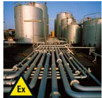
Typical hazardous gas areas are found in the chemical industry, for example in gas and petroleum processing.
